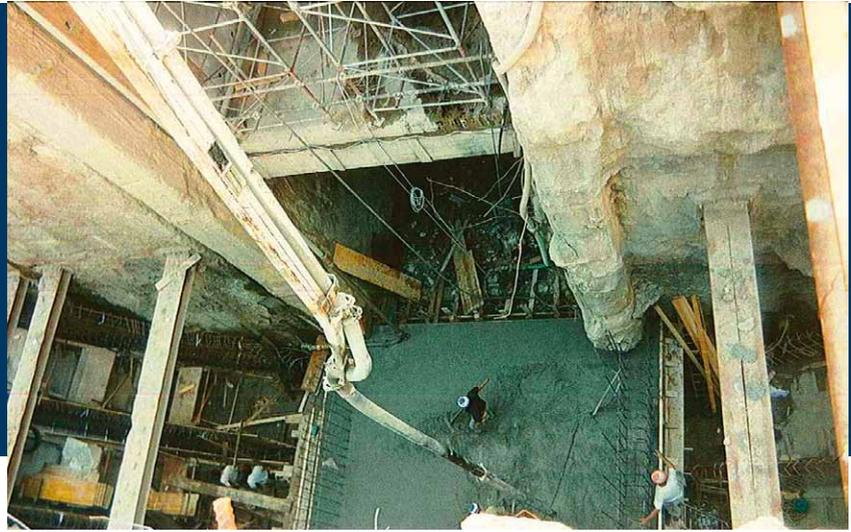
Small diameters for a small Cipa. In 1992, we started working on the extension of line A of the Rome Underground, building two sewer lines for a total length of about 100 metres, with an excavation cross-section of only 4.5 m<sup>2</sup>, hand-made, and ancillary works.
