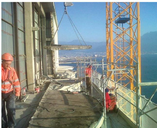
*The subsequent controlled demolition in elevation involved the walls of the cells and the parts over the slabs, using scaffolds and cranes.*
