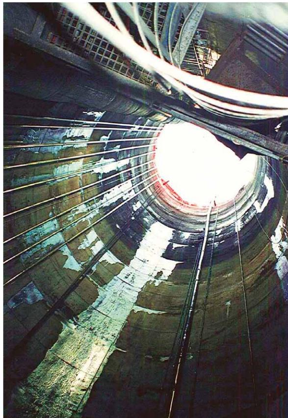
*first time in Italy, was carried out with the freezing technique, similarly to the connection adits to the line. The connection adits to the line tunnels, respectively 5 and 13 metres in length, had an excavation cross-section of 11 m<sup>2</sup>.*
