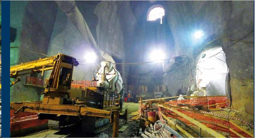
*directional scaffolding was erected ad hoc, with irregular geometries adapted to the cavity's morphology, making it possible to reach these heights. The operations were completed with the laying of welded wire mesh and shotcrete.*
