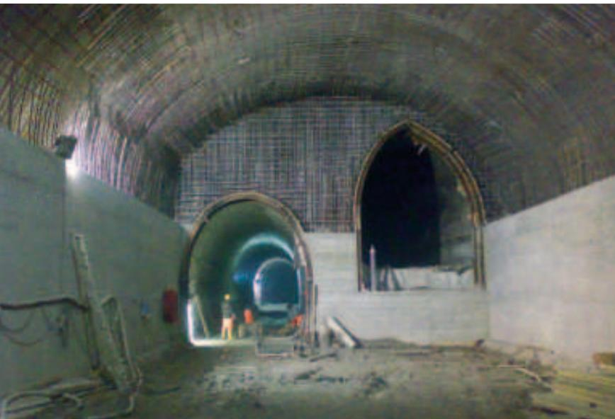
*The excavation proceeded in current section, covering the partial section with reinforced concrete before the start of the subsequent bench phases.*
